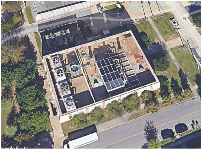
Equipment on roof
