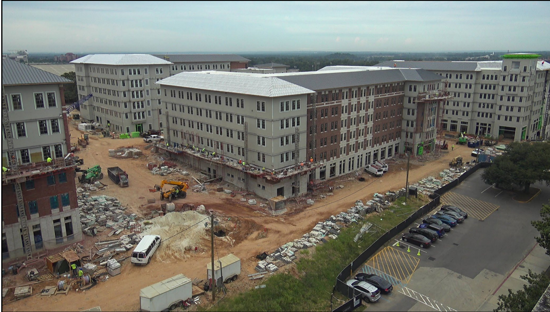
Current view from Bates House. All buildings “dried-in”, masonry veneer ongoing.
